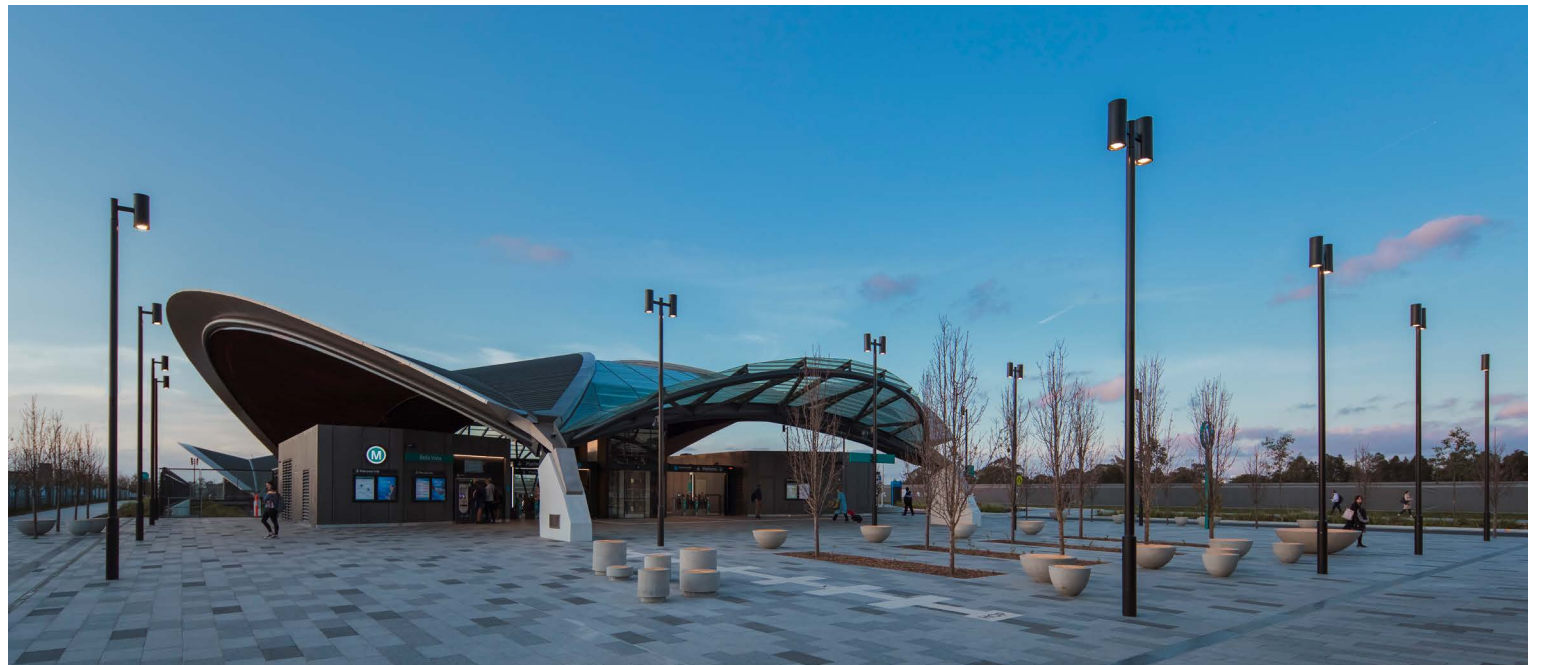
TANGO POSTTOP LUMINAIRES INSTALLED AT NORTH WEST SYDNEY METRO STATION NSW
