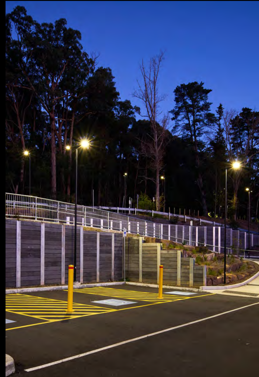
BILLUND STREET AND AREA LUMINAIRES INSTALLED AT PUFFING BILLY CARPARK VIC
